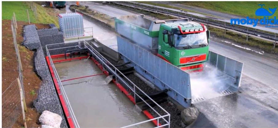
Figure 5.1 Example of Wheel Washing System
