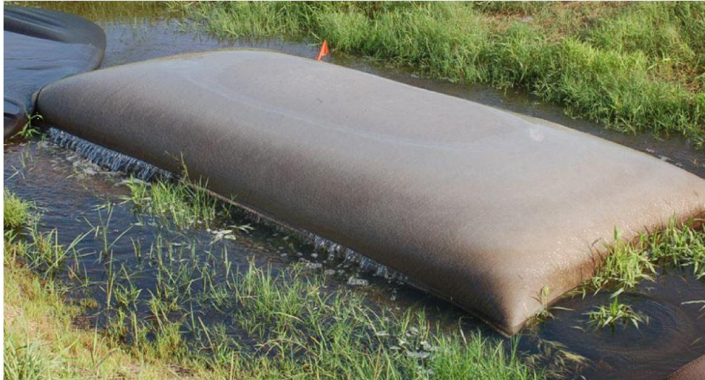
Figure 5.4 Example of Silt Dewatering Bag
